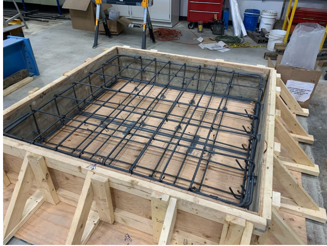
Figure 5.3 – Reinforcement cage prior to embed placement and concrete pour (lifting hooks not shown).
