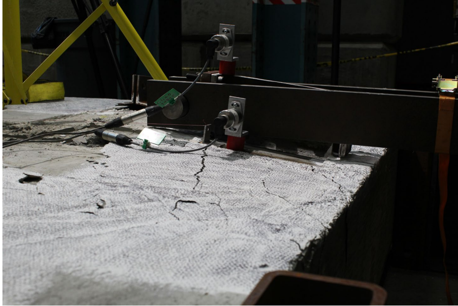
Figure 6.6 – Side view of ST-175 P at peak displacement, displaying a combination of tension and shear breakout, or a pryout style failure
